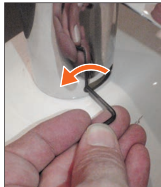
ATM606/607 ISOLATION VALVE IMAGE 56
